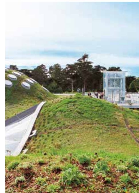
Living roof atop California Academy of Sciences
